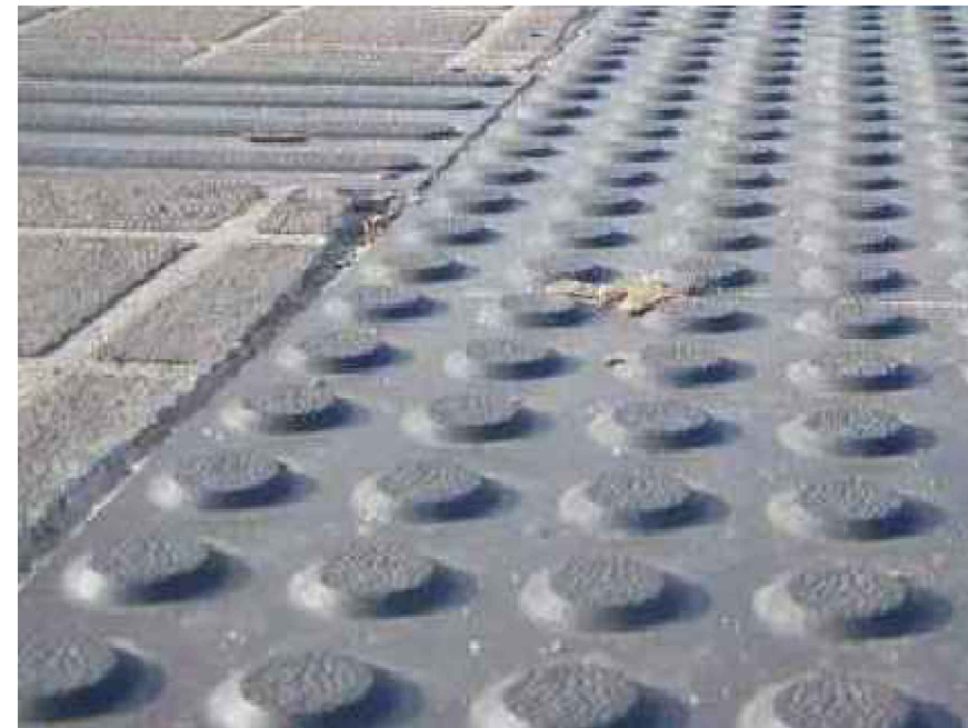
REFERENCE IMAGE TYPICAL BLISTER PAVING
