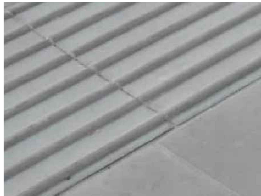
REFERENCE IMAGE TYPICAL TACTILE CORDUROY PAVING
